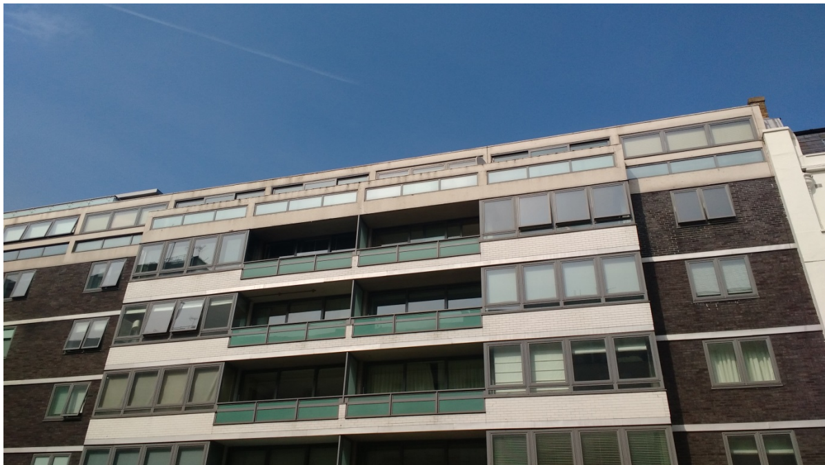
View of Flat 25 from Lowndes Street
